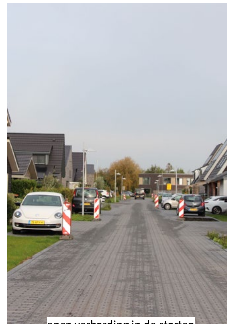
open verharding in de starten
